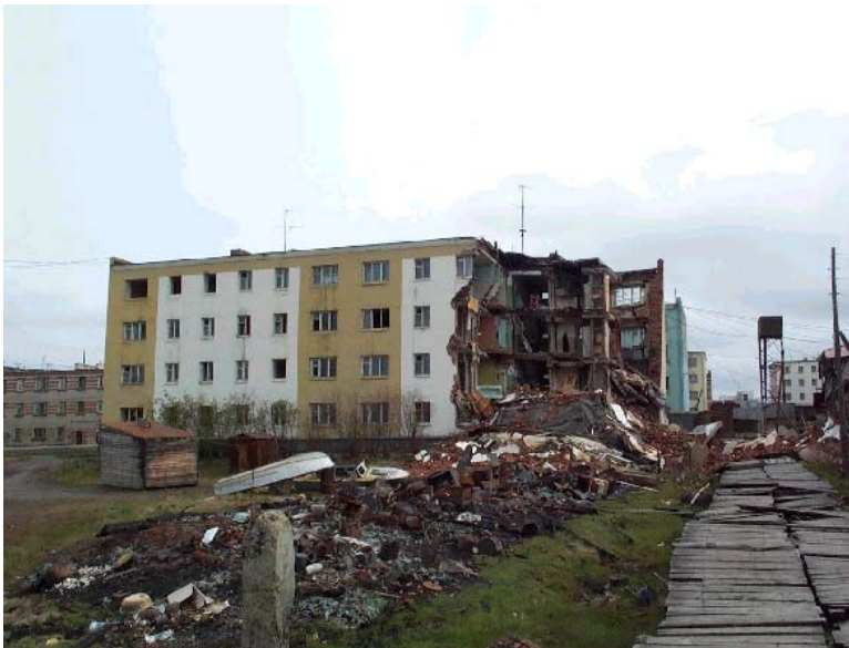
Figure 16: Uneven settling due to permafrost thaw destroyed this apartment building in Cherski, Siberia, which occurred only days after the appearance of the first cracks (photo: Vladimir Romanovsky).
