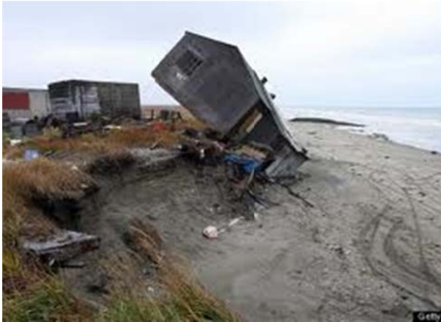
Figure 18: Coastal erosion of permafrost resulted in the complete destruction of this house in Shishmaref, Alaska (photo: TBD).
