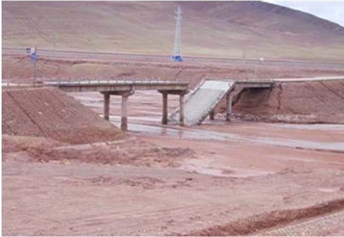
Figure 17: Permafrost thawing near the base of the support pillars caused this bridge on Qinghai-Xizang Highway in Tibet to collapse (photo: Tingjun Zhang).
