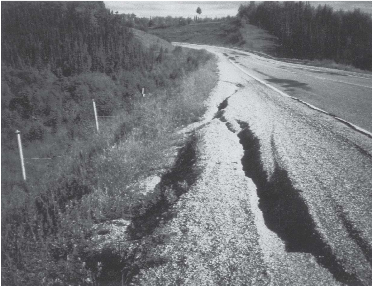
Figure 13 Longitudinal cracks in a road embankment near Fairbanks, Alaska. Snow removal during winter produces a berm along the shoulder and slope of the embankment that warms the underlying ice-rich permafrost, causing it to thaw and settle. Settlement under the shoulder and slope causes the edge of the embankment to tilt outward, putting the top surface of the embankment in tension, which eventually results in cracks. Patches (darker asphalt) in the pavement are a result of two long cracks and the guardrail on the far side of the road has sagged as a result of the thaw settlement. (Photograph by T. E. Osterkamp.)
