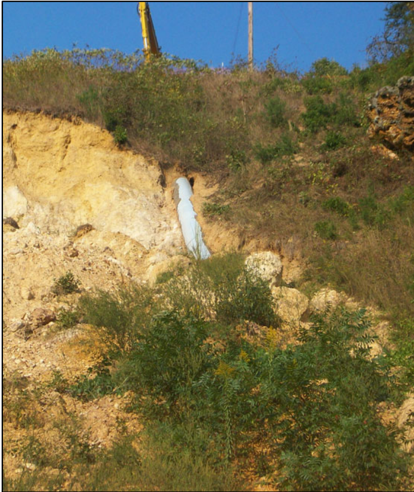
Figure G-1. Pipeline exposure caused by mass movement of soil on steep terrain. (source: Jones Contractors, Inc., 2014).
