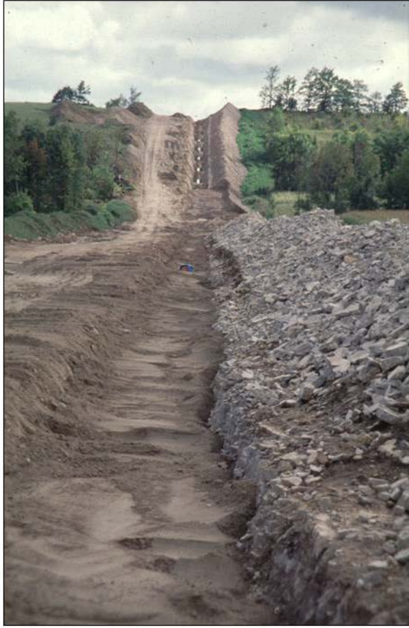
Figure N-2. Back-filling of pipeline trench in variable terrain ( foreground - shallow to bedrock; background - steep topography over drumlin) (photo: R.A. McBride).
