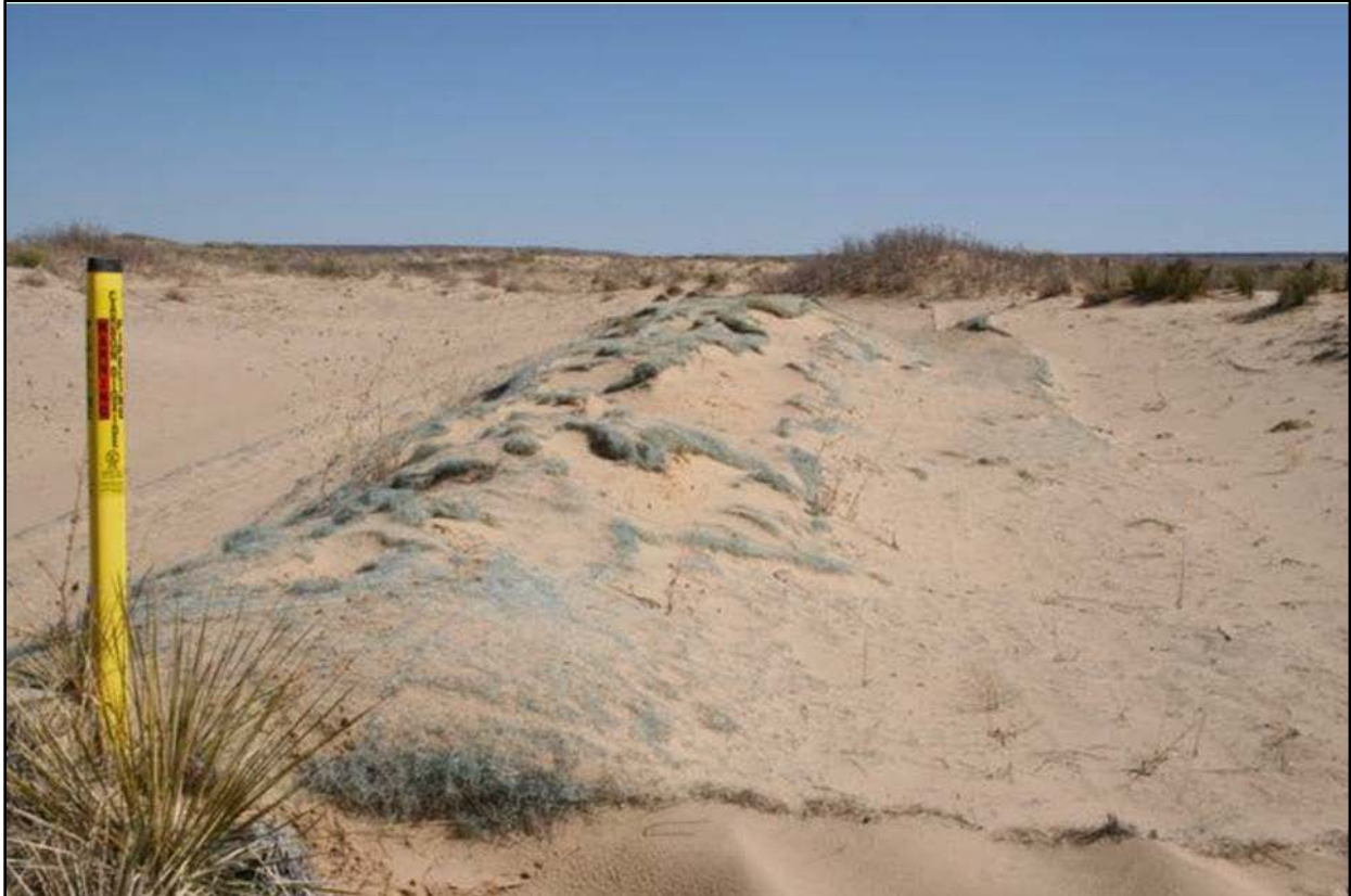
Figure G-4. A dryland blowout caused by wind erosion on a pipeline ROW in southeastern New Mexico, with a damaged geotextile erosion mat emplaced only one year prior. (after Peterson, 2013).
