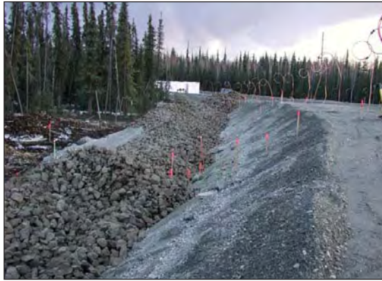
Figure 2. Shoulder installation.
