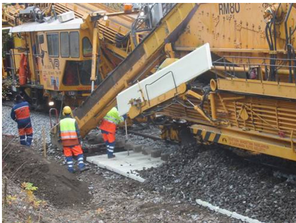
Figure 6 Installation of XPS frost insulation boards during ballast cleaning
